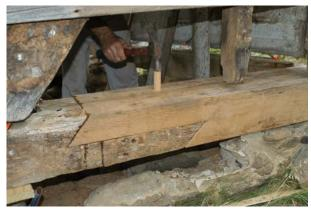
Mike Adams is hammering a peg into the a perfectly scarfed sill joint in southeast corner of the house.
