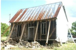
The Hollow on June 20, 2005. Note the foundation stones stacked up on the north side and the hole underneath the house.
