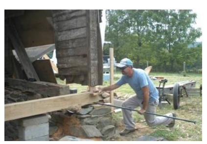
Mike has to lift the west end while the timber is being driven toward him. The photograph on the right shows the sill where Mike wants it to finish the ends of the studs.
