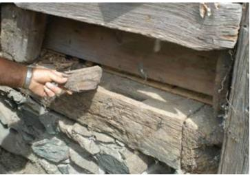
During inspection of the front portion of the west side chimney sill, the period-one carpenter's patch of a mistakenly-placed downbrace mortise was discovered. The infill block of wood was just set loosely into the mortise. Also of interest, there should be a stud between the corner post and the left downbrace as there is at the north side of the chimney, but there is no evidence of a smaller mortise for one.
