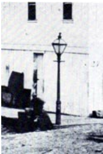
A better view of one of Little Rock's gas streetlights, a simple glass lantern atop a cast iron post. The lamp-lighter used a ladder, steadied against the crossbars, to climb up, open the gas valve and light the lamp each evening, repeating the process each morning to turn the lamps off.
