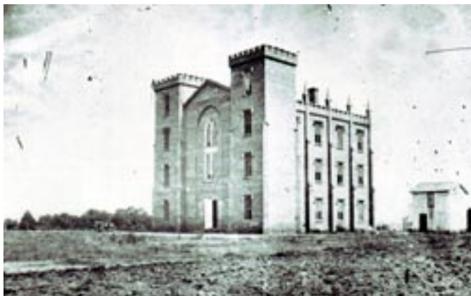
Only what was planned as the east wing of the academic buildings of St. John's College was ever constructed. The school opened in 1857, but closed in 1861 when the student body enlisted in the Confederate Army. Used by both sides as a hospital, in January 1864 the lawn shown here in front of the building was the site of the execution of David O. Dodd.
