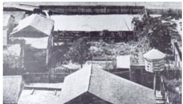
This 1863 view of a back yard in the residential area shows an important feature of Little Rock homes during the times... the privy, or "necessary house." Here two adjoining homes have their privies located side by side along the back fence line. Little Rock had no sanitary sewers. An 1833 city ordinance required persons owning or occupying a lot where a "necessary house" was located to keep "the same in a neat and clean manner." Contracts were awarded for the cleaning of privies and the removal of "night soil," and the city ordinance further required that privies be equipped with watertight boxes easily accessible to the privy-cleaner. Note the gardens and sheds visible, as well as the purple martin house at the right... to help on mosquito control!
