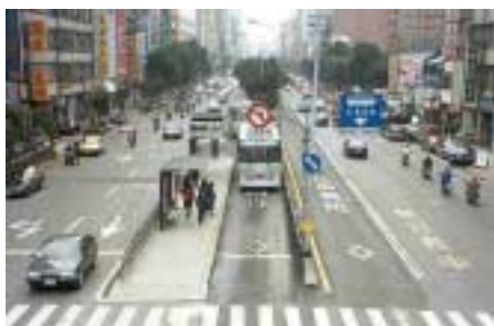
Taipei's successful new bus lanes in the centre of the street. Photo: Barter
