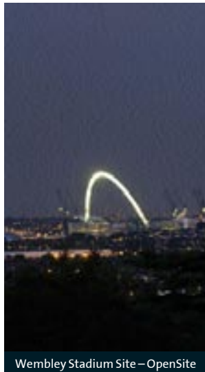
Wembley Stadium Site - OpenSite
